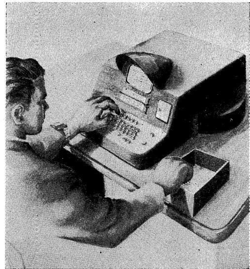
Fig. 7—Flight data-entry equipment.
