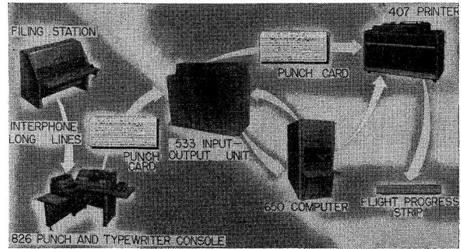
Fig. 5—IBM 650 air-traffic control operation.
