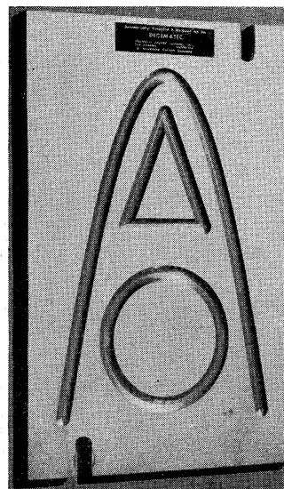
Fig. 9—Geometric contours produced by model 120 DIGIMATIC computer.
